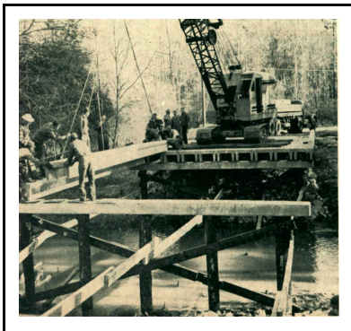
Figure 18. The state's first prestressed concrete double T bridge under construction in 1955. Source: Carolina Highways , March, 1955.
