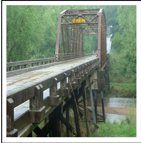
Figure 8. 1922 thru truss span relocated to Union County in 1962 as part of new bridge over the Tyger River. Transystems.
