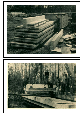
Figure 17. Precast slab units stacked at casting yard prior to shipment to bridge site and units being hoisted into place. Note integral curb cast into top beam. Carolina Highways , Oct., 1950.
