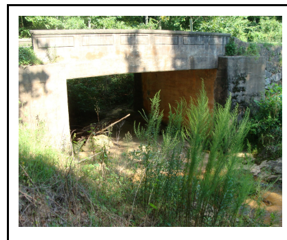
Figure 13. The 1910 slab bridge on Old Buncombe Road near Travelers Rest is one of the oldest reinforced concrete bridges in the state. Transystems.
