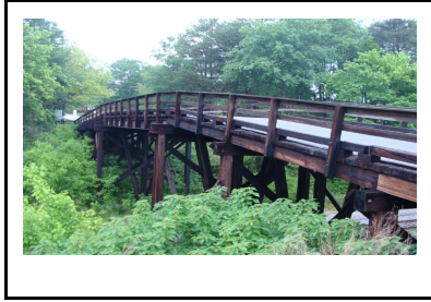
Figure 2. Typical timber stringer bridge construction with timber railings and timber pile bents. This bridge dates to ca. 1918 and crosses the Southern Railway in Spartanburg County.
