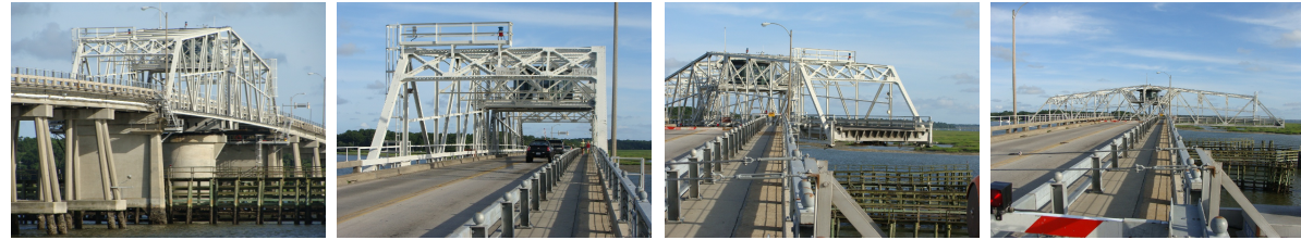
Figure 20. US 21B over Beaufort River 1957-1960 swing span bridge showing elevation of movable span, roadway through the movable span, movable span rotating open, and bridge in the open position to allow passage of marine traffic. TranSystems, 2013.
