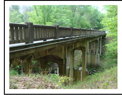
Figure 1. Old SC 7 over Shanklin Creek Bridge in Abbeville County stands as one of the complete early examples of the state standard design T beam bridge. It was constructed in 1924. Transystems.
