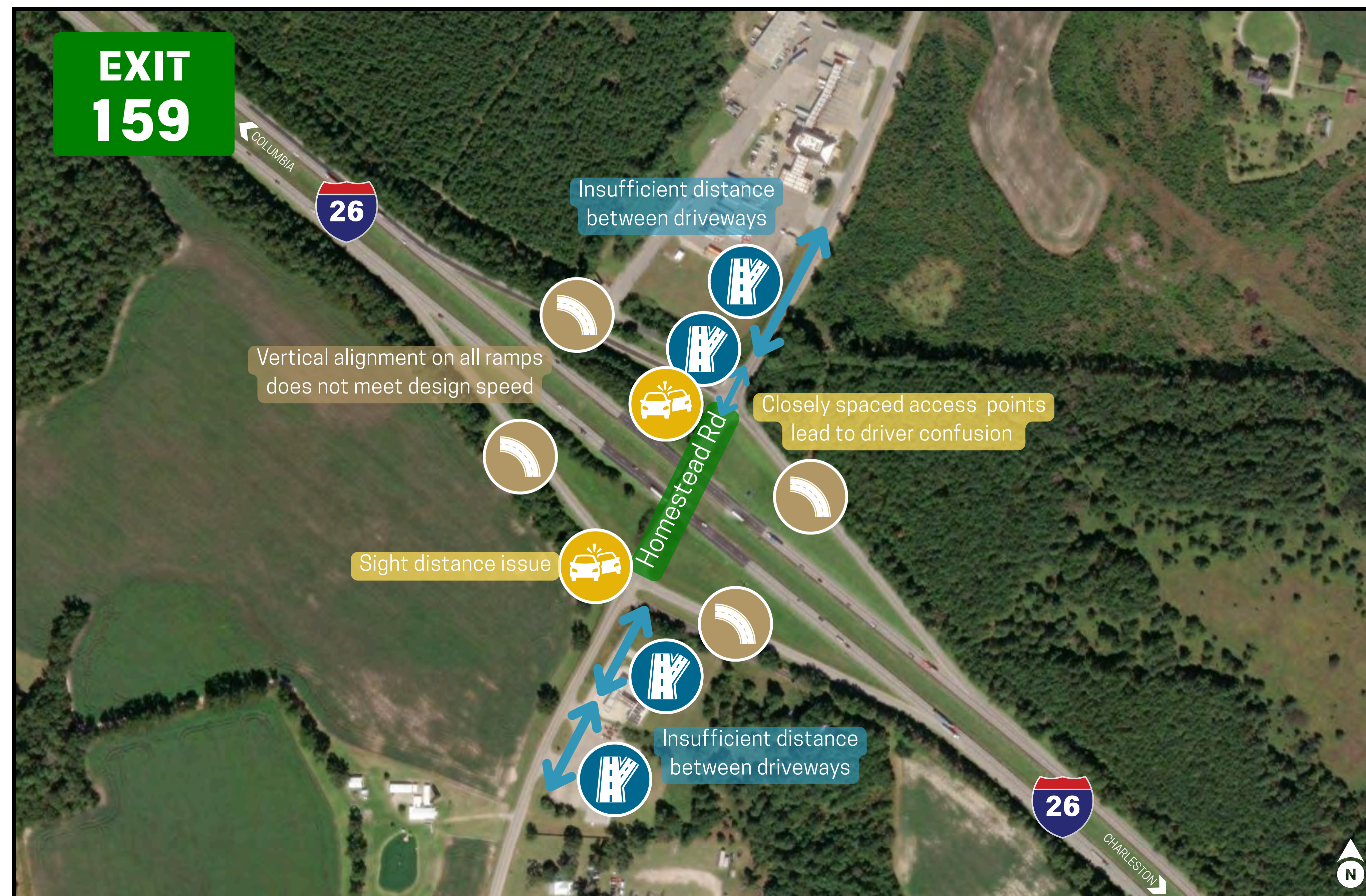
Exit 159 (S-36/Homestead Rd)
